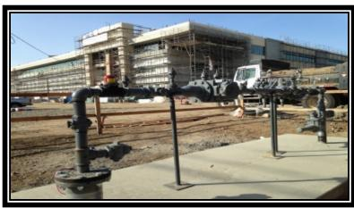
The gas meter was relocated next to the utility yard and gas line connected to the buildings on campus.
